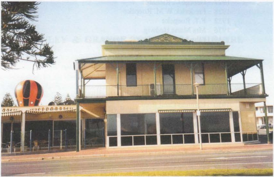
Henley Hotel showing dining area and still-enclosed verandah, 2006; the cast-iron balcony brackets have gone.
