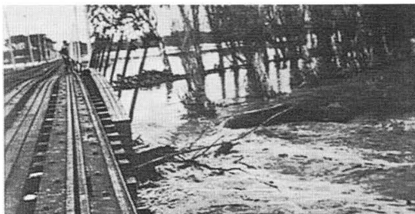
Above: Flooding under the tram viaduct through Reedbeds, 1917. Below: Flood in the Flinders Park area, 1931, with tops of greenhouses visible. (Photos courtesy of State Library of South Australia)
