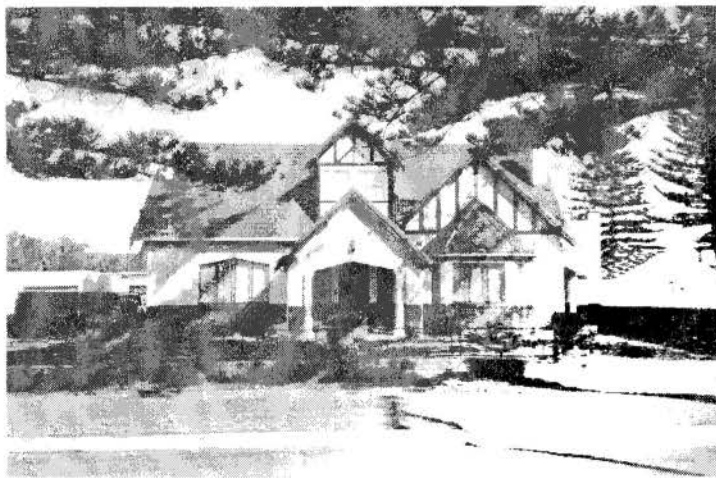
House, 9 Rockingham Street, West Beach, 2000
