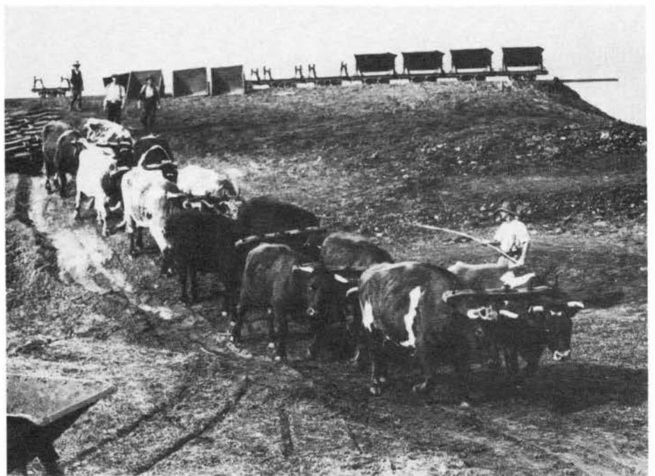
Bullock team working on construction of Torrens outlet, May 1937
