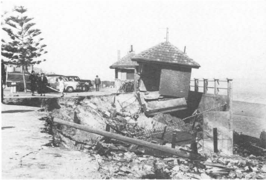
Storms frequently destroyed 'improvements' made along the foreshore. The storm on 18 May 1953 caused considerable damage, with gusts over 100km/h being recorded. Location: Henley Beach Road.
