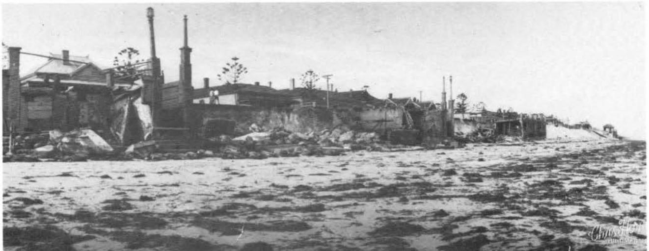
Storm damage, May 1953
