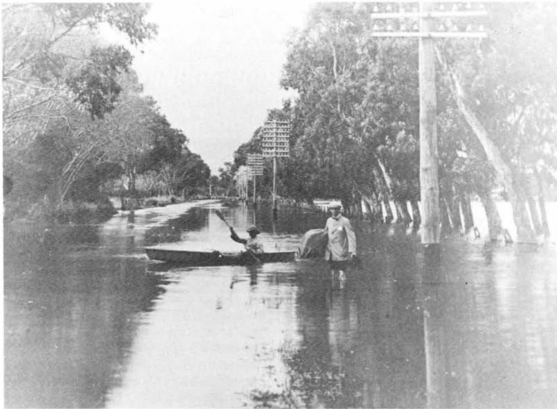
Flooding on the Henley Beach Road, Fulham, west of Tapleys Hill Road
