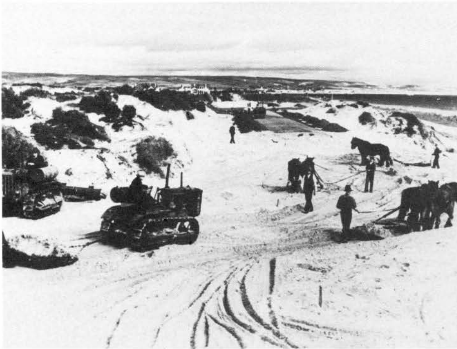
Work on the Torrens outlet 1937. Some of the original houses at West Beach are visible in the centre.
