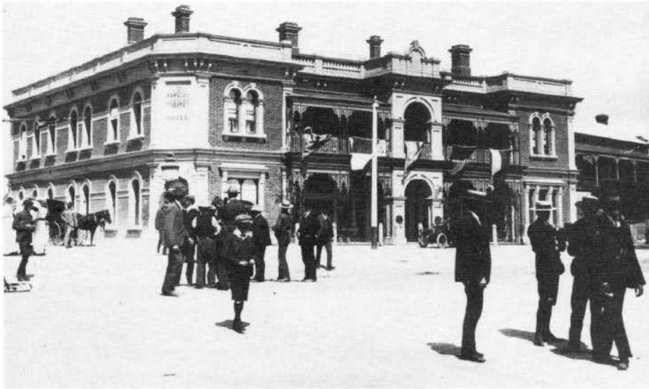
Ramsgate Hotel c1904-7, before balcony was added.
