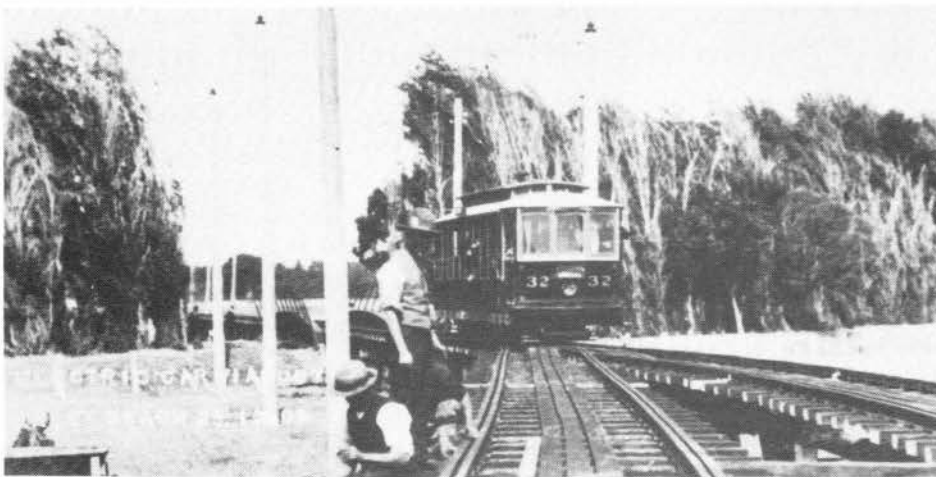
Opening day of the newly electrified tramway to Henley—'toast rack' tram No 32 on the viaduct over the reedbeds, 23 December 1909.
